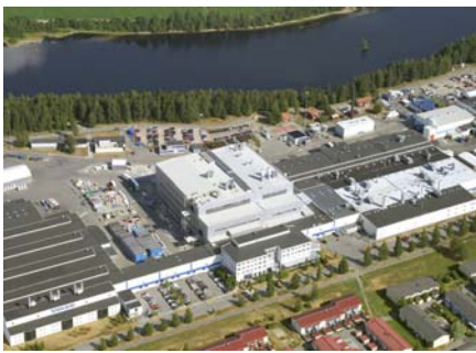
Volvo Trucks Operations site in Umeå
